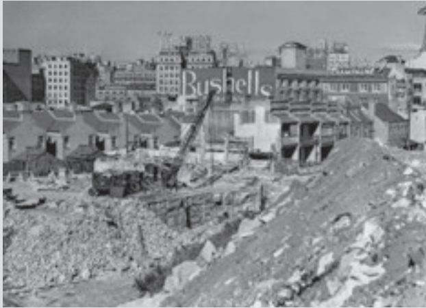
FIGURE 6 Excavation through The Rocks for construction of the Cahill Expressway's southern approach to the Sydney Harbour Bridge in 1955.
